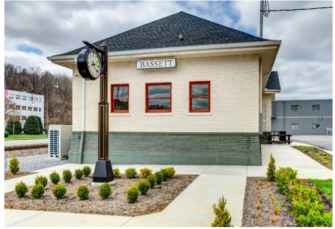
An example of clock tower improvements to the Bassett, VA depot, including a clock and public gathering area
