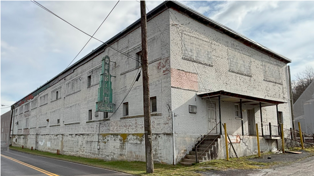
Existing Façade: 1610 Riverside Drive
