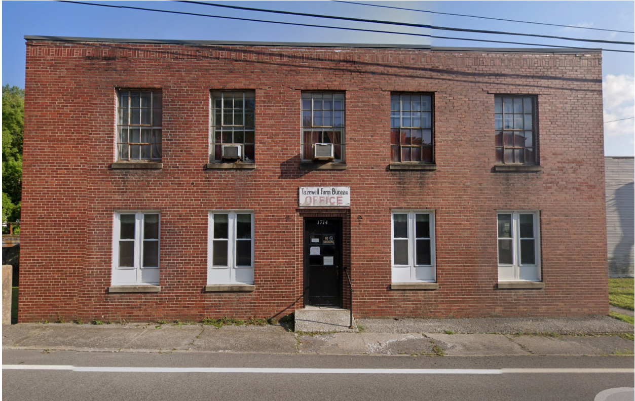
Existing Façade: 1714 Riverside Drive
