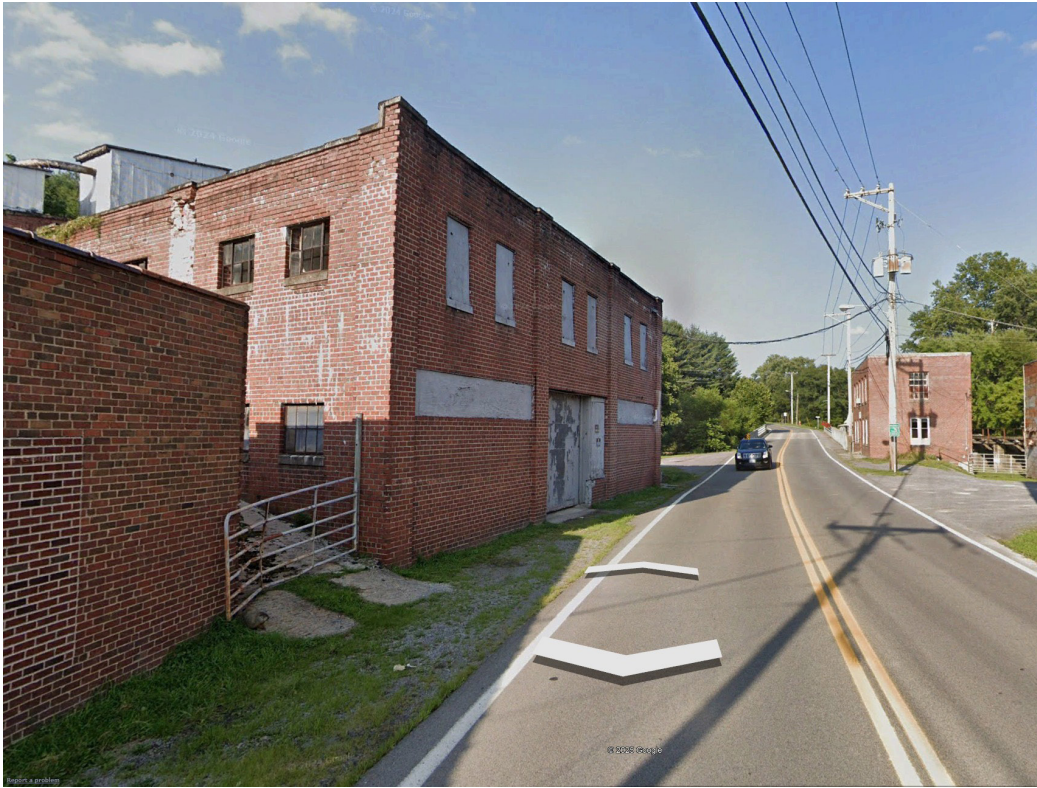
Existing Façade: 1693 Riverside Drive (South and West)
