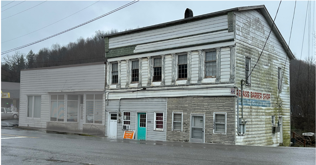
Existing Façade: 1339 Tazewell Avenue
