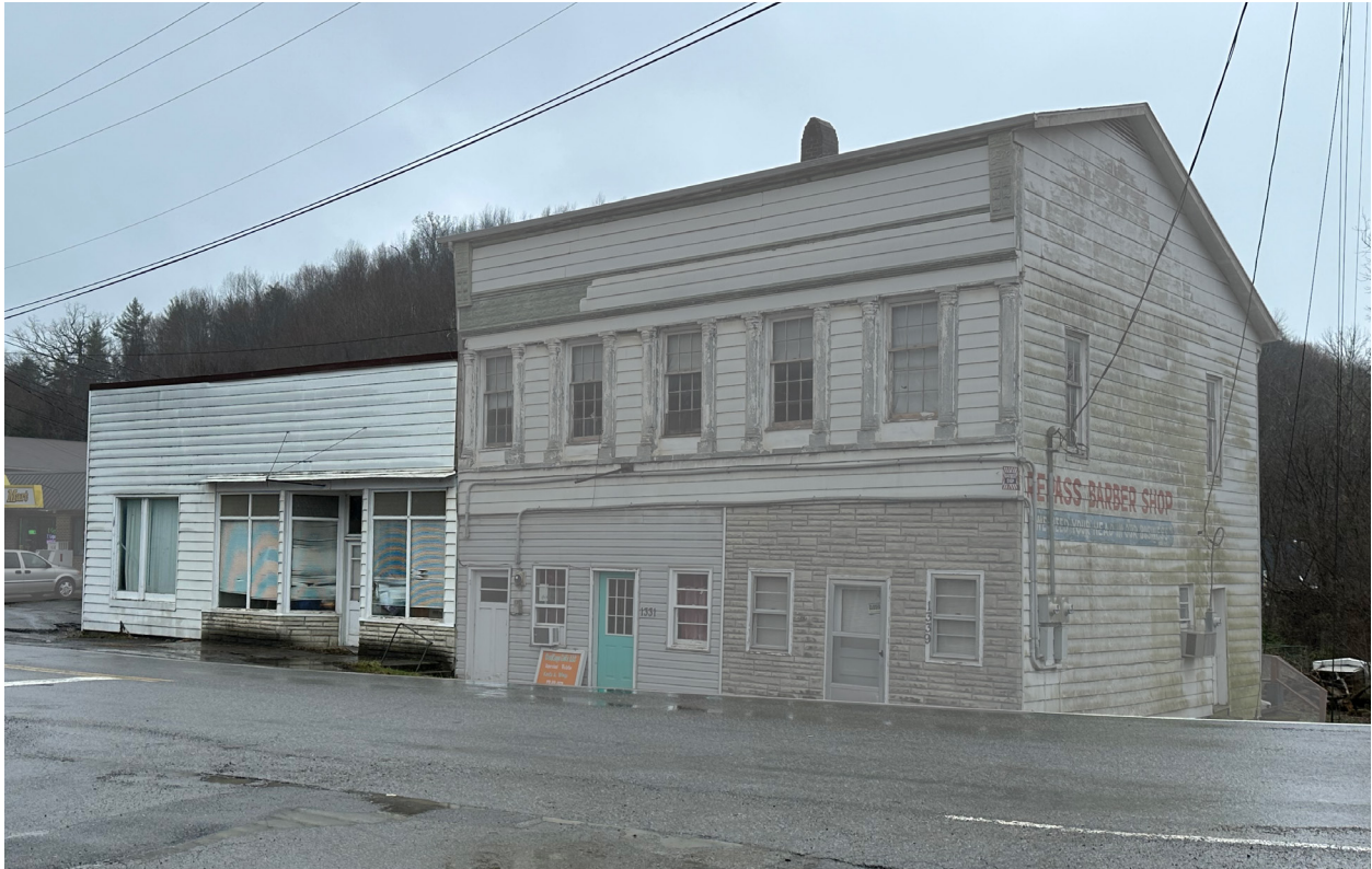
Existing Façade: 1331 Tazewell Avenue
