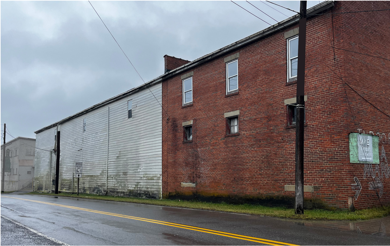
Existing Façade: 1532 Riverside Drive
