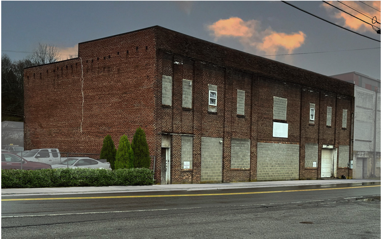
Existing Façade: 1616 Riverside Drive
