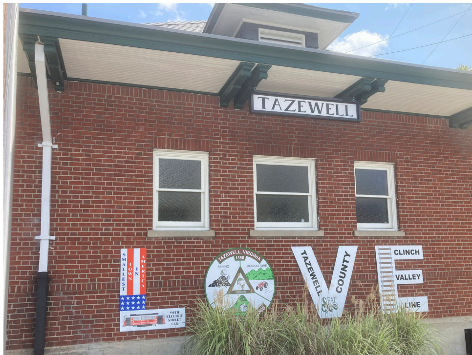
Tazewell Train Station and Visitor Center
