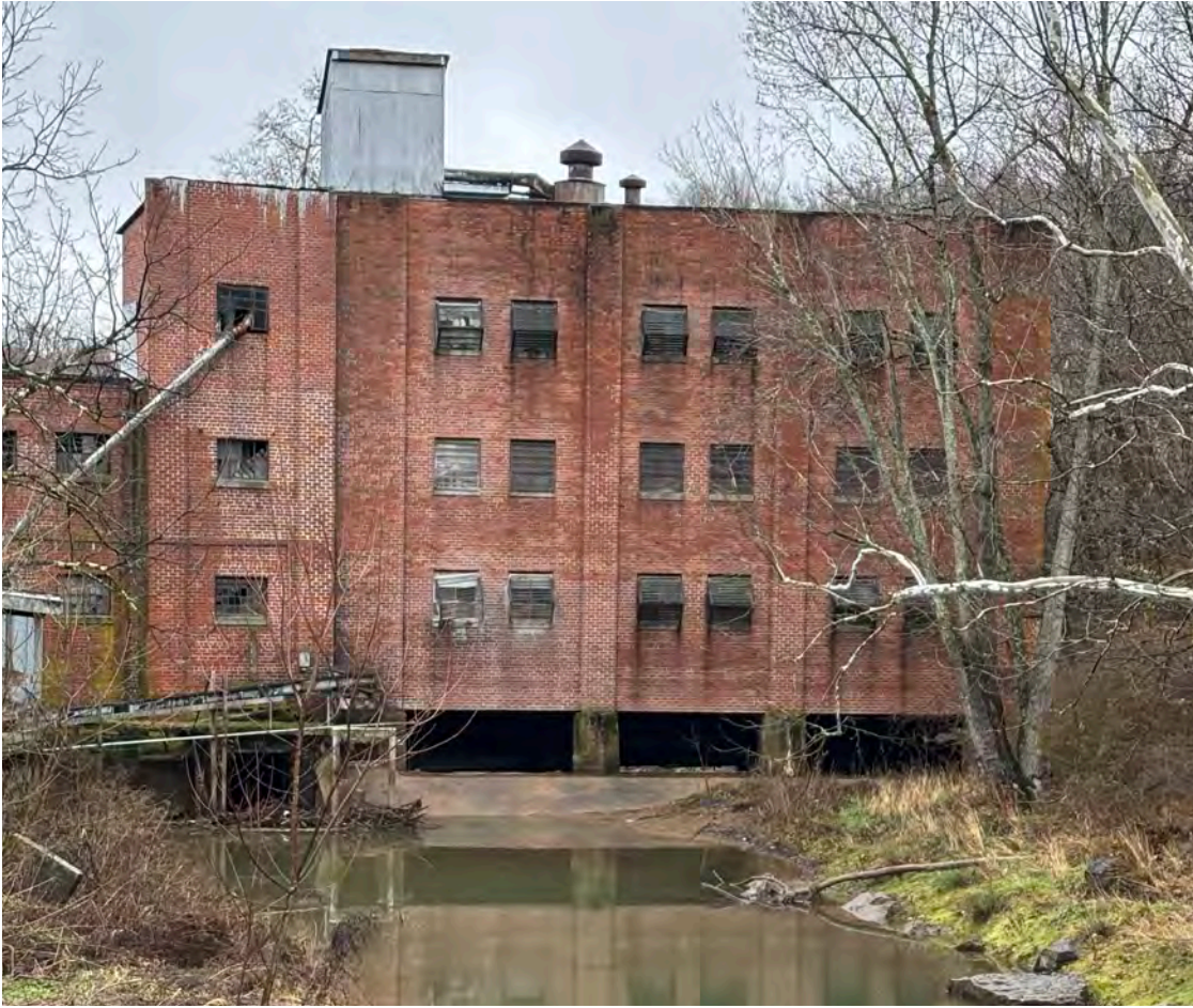
Existing Façade: 1693 Riverside Drive (East)
