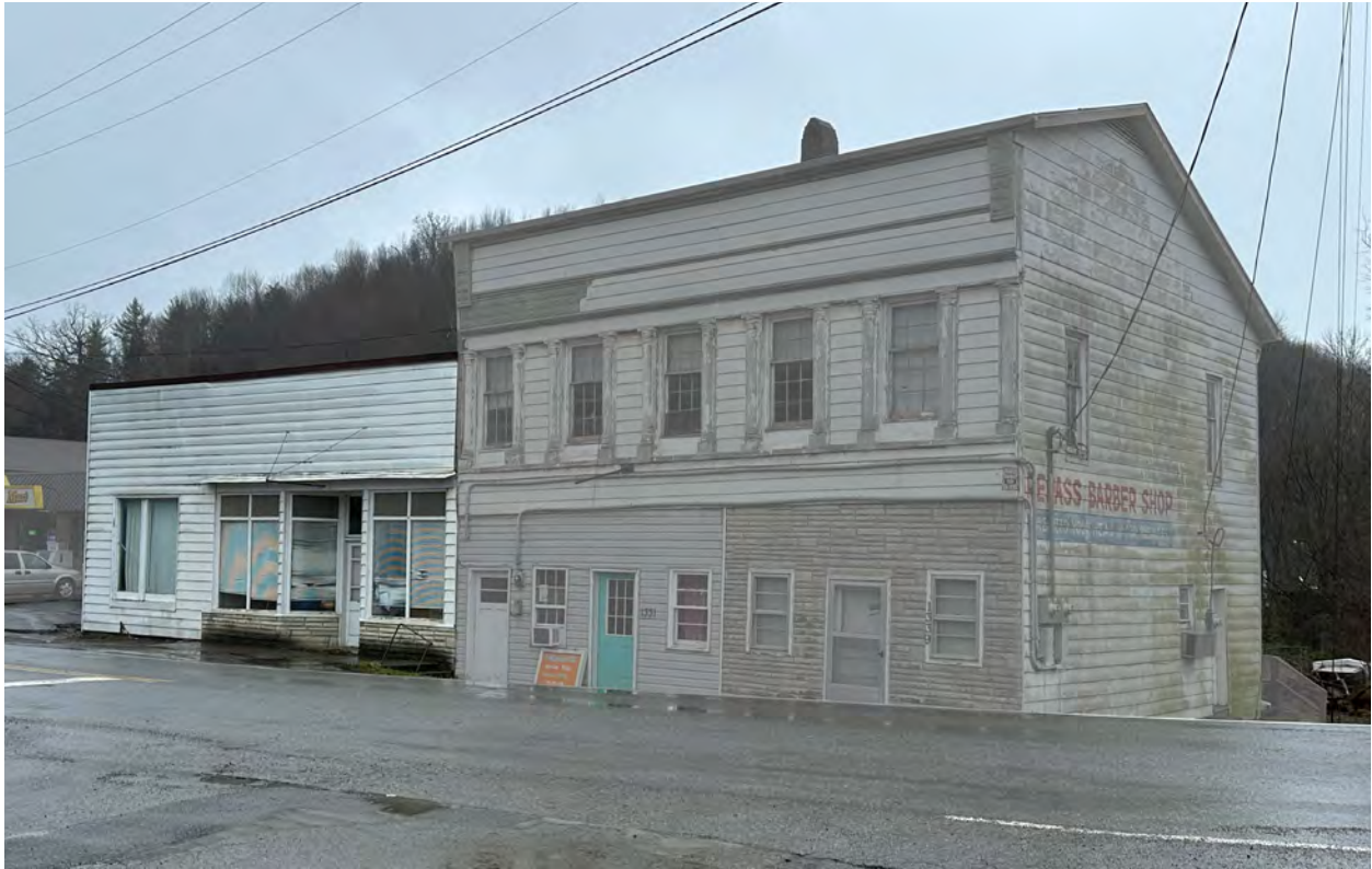
Existing Façade: 1331 Tazewell Avenue
