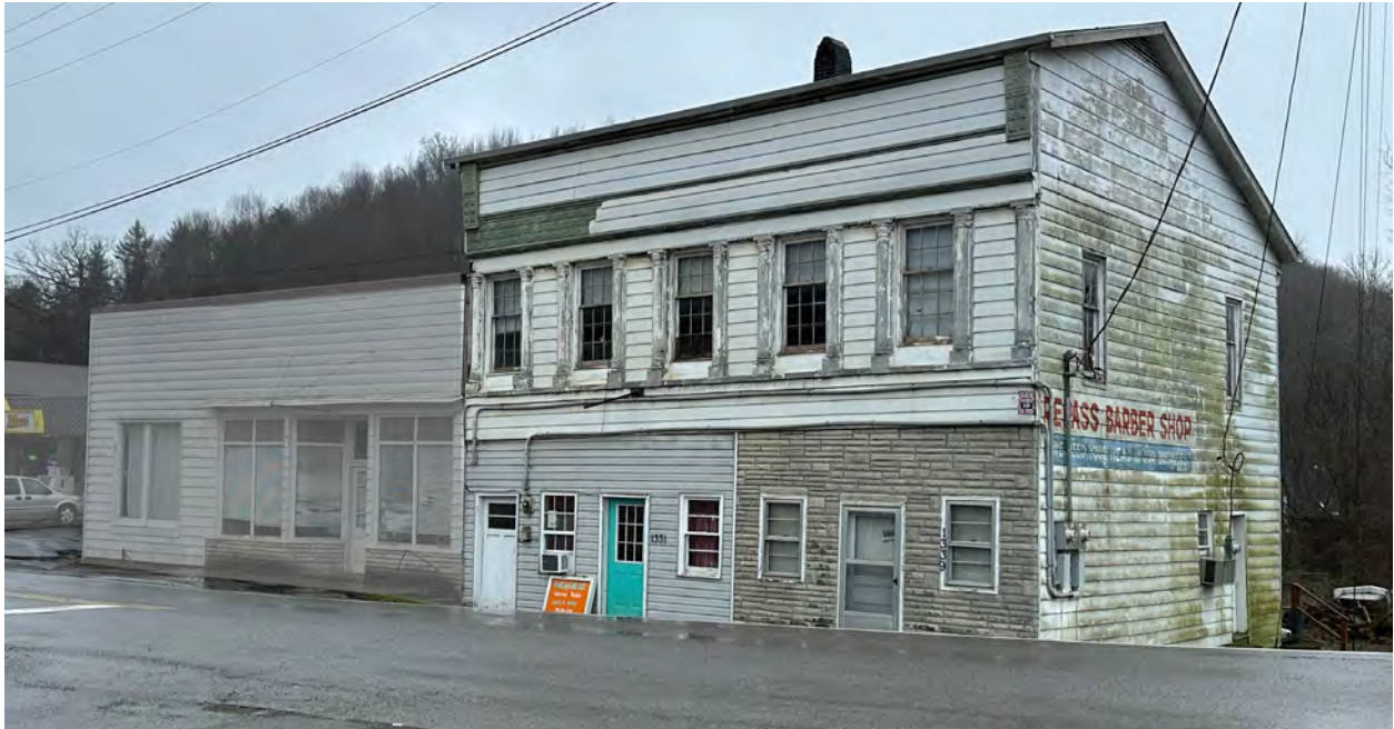
Existing Façade: 1339 Tazewell Avenue
