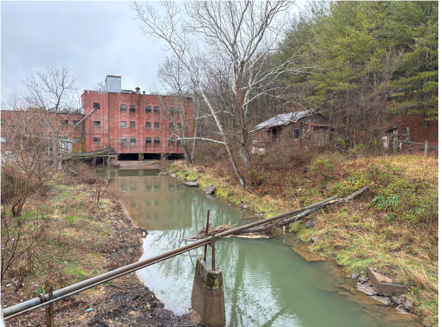
Tazewell's mill over the Clinch River.
